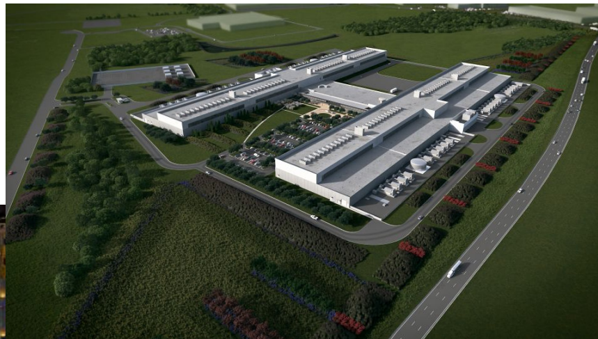
facebook 2nd datacenter
